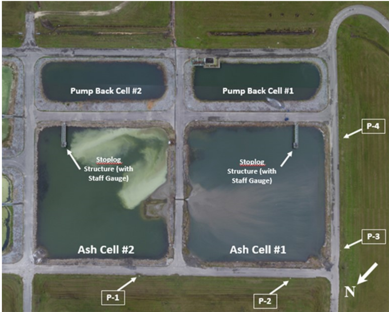
Figure 1. Aerial View of the CCR Surface Impoundment System (IWCS 2016)
